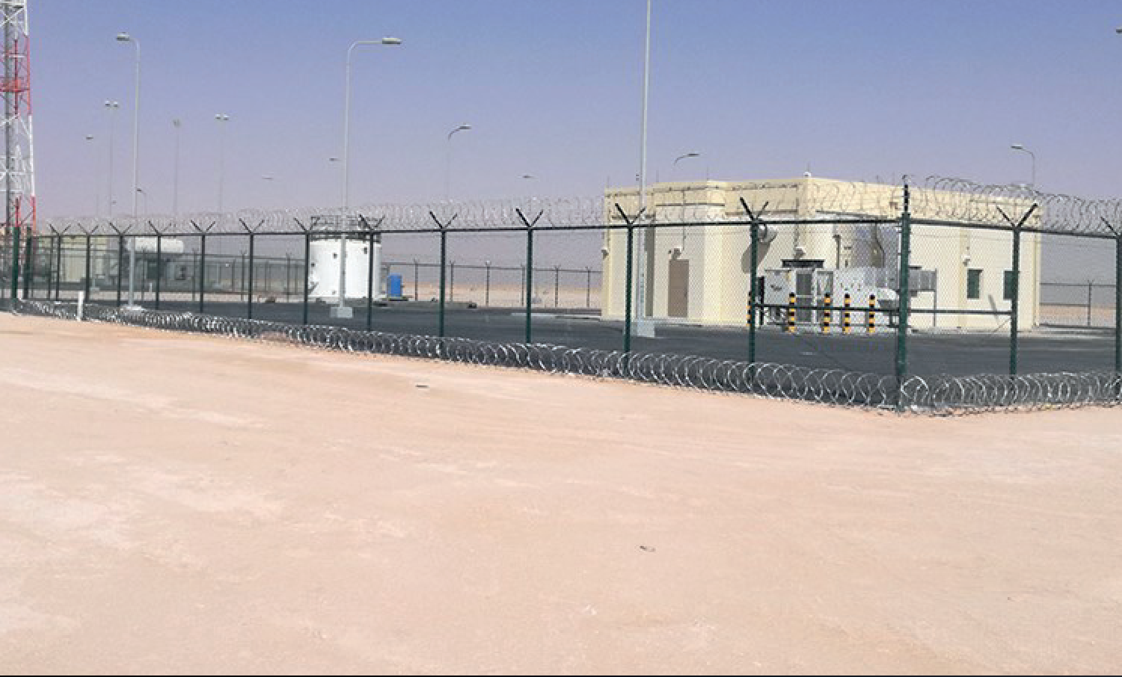
HARADH SATELLITE FIELDS CONSTRUCTION PROJECT
